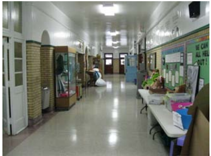
Surface Mount 1x4 Direct Fluorescent Light Fixtures
