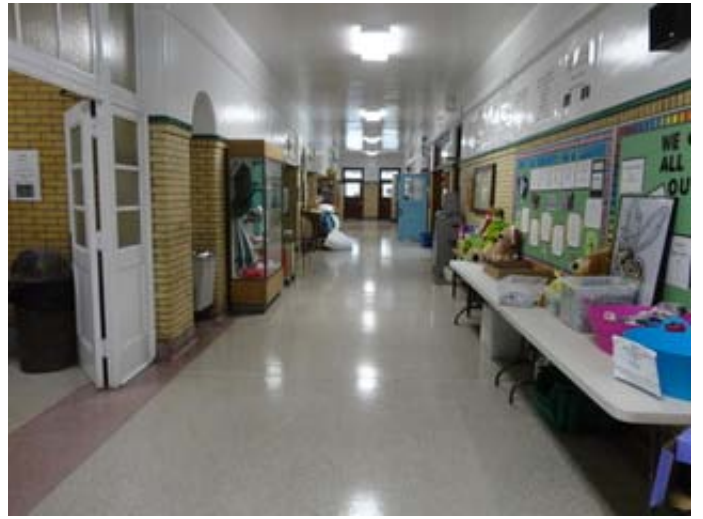
Typical Corridor Finishes in 1918 Original Construction
