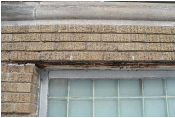
Typical Lintel in 1918 Original Construction
