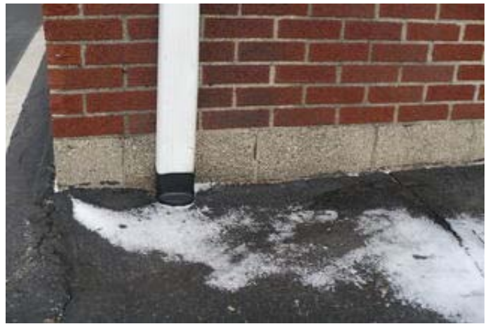
CMU Foundation Wall of the 1956 Music Addition
