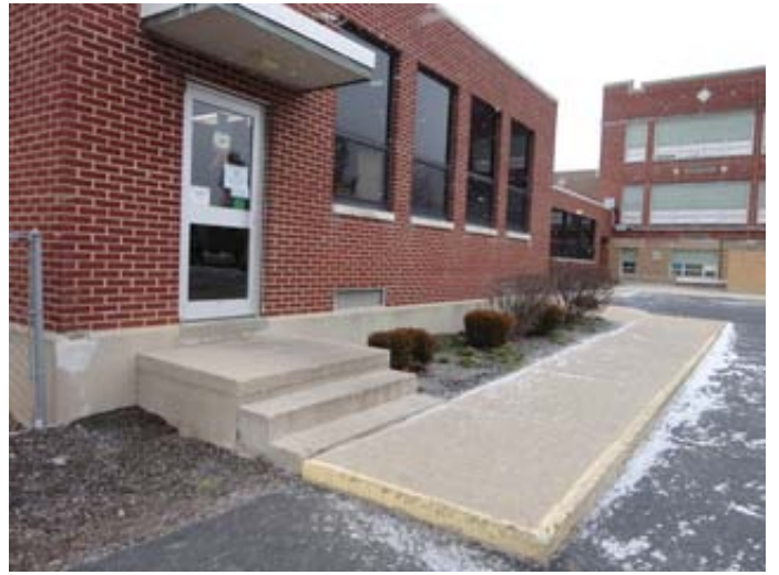
Steps and Sidewalk
