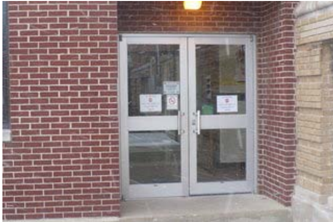
Typical Entrance Doors in 1951 Addition
