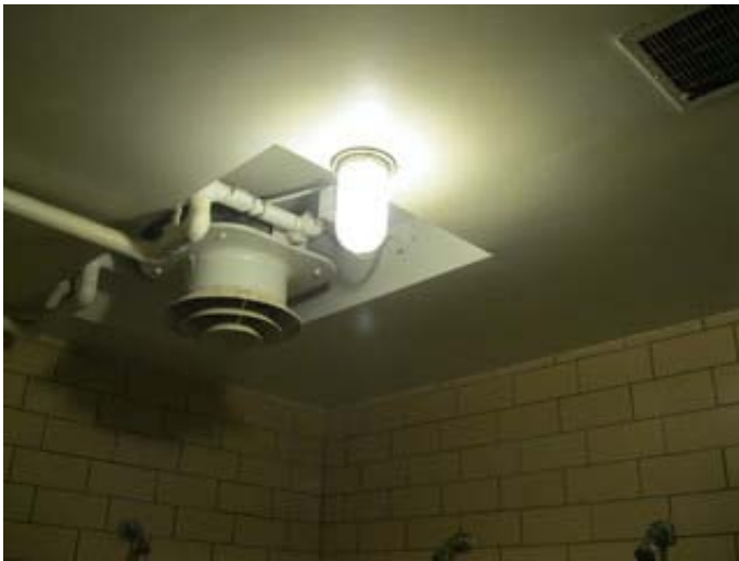
Surface Mount Incandescent Light Fixture
