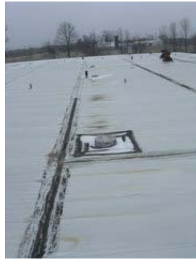
Typical Sheet Steel Roofing
