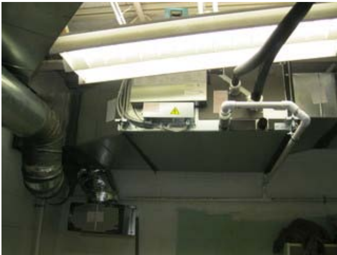
Mitsubishi Ceiling Concealed Indoor Unit/Ducted Fan Coil
