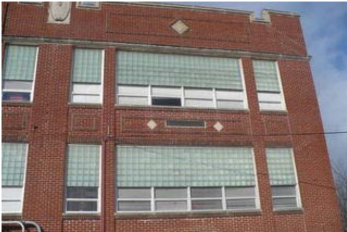
Typical Windows in the 1918 Original Construction
