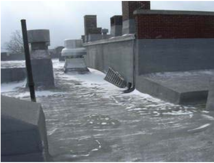
Typical Foam Roofing
