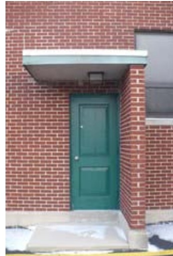
Typical Wood Exterior Door at the 1951 Addition
