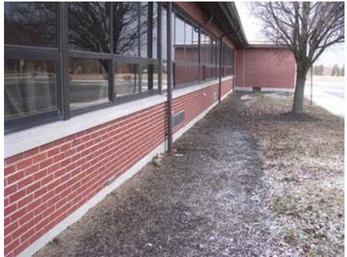
Typical Gutter and Down Pipe Condition
