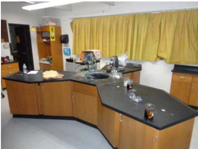
Asbestos Laboratory Tops
