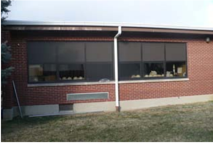
Typical Classroom Window of 1964 Addition
