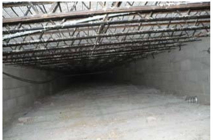
Crawl Space of the 1964 Addition
