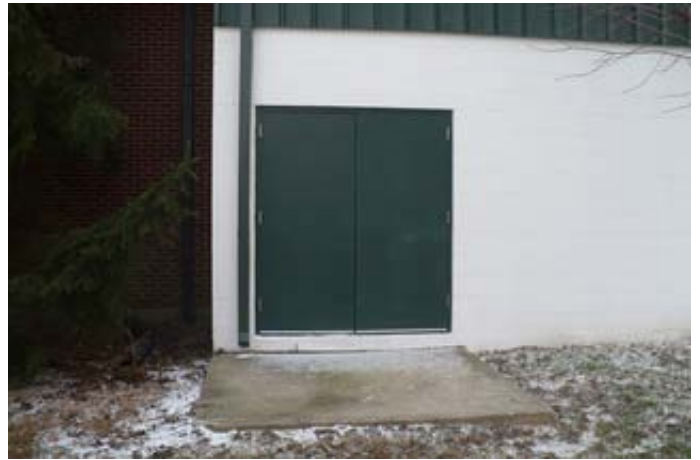
Exterior Doors of the 1999 Addition
