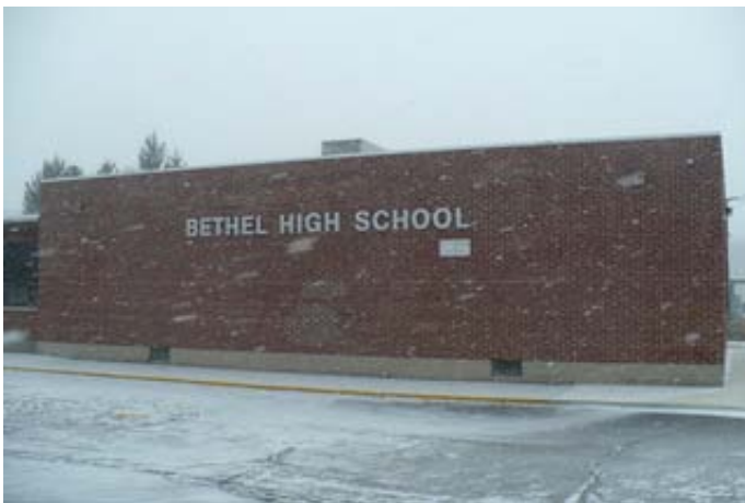
Brick Masonry of the 1964 Addition
