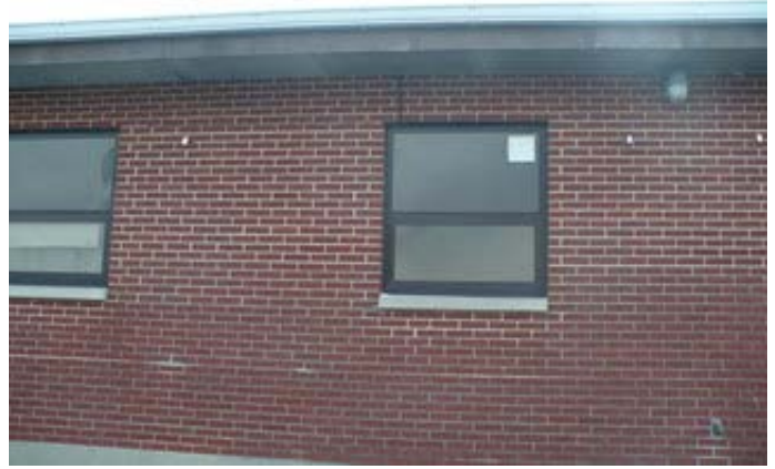
Typical Prep Room Window of 1964 Addition
