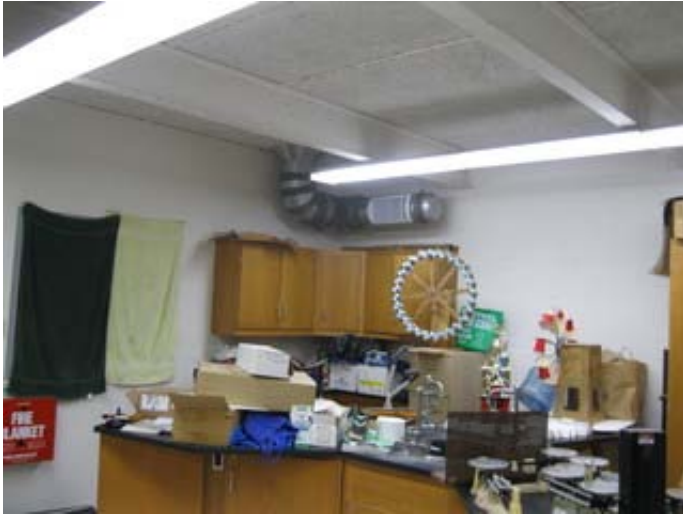
Typical 1964 Addition Steel Roof Framing and Tectum Panel Roof Construction
