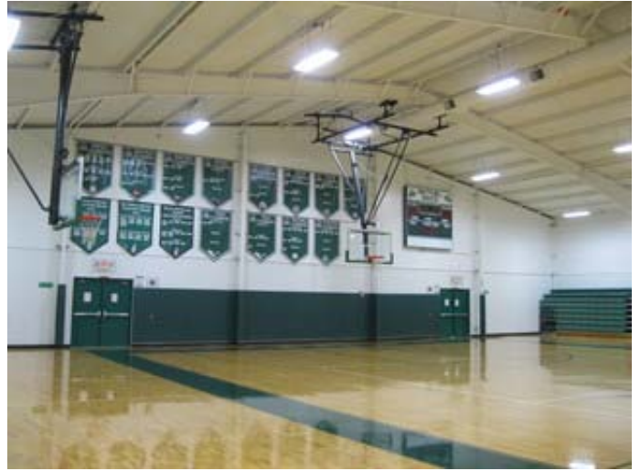
Typical 1999 Addition Steel Frame and Tectum Deck Construction
