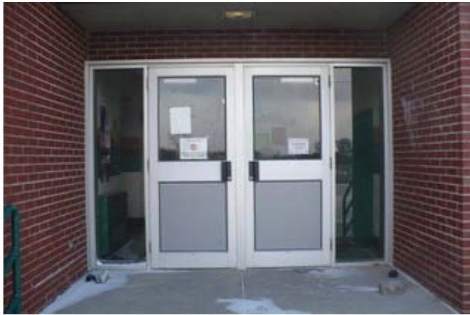
Entrance Doors of the 1964 Addition
