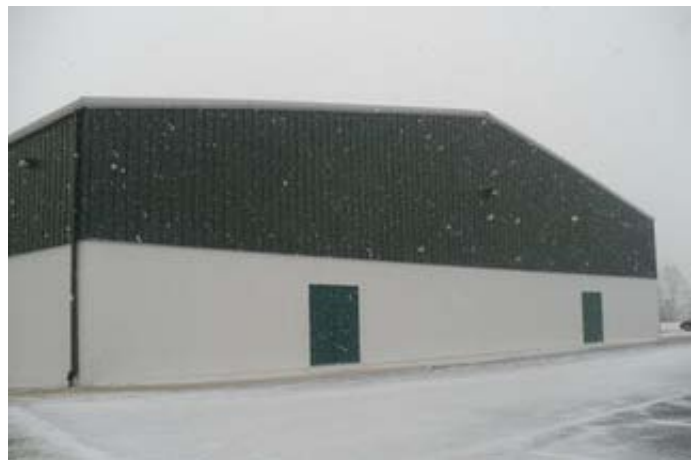
CMU and Metal Siding of the 1999 Addition
