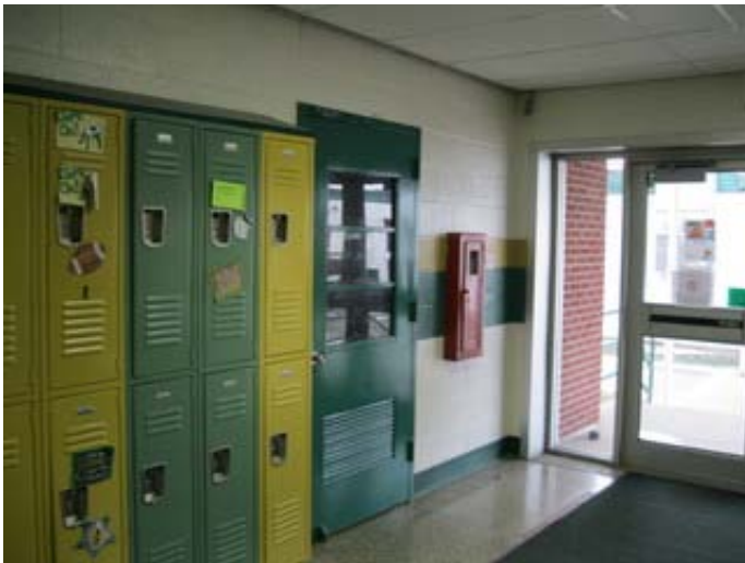
Typical Fire Extinguisher Cabinets
