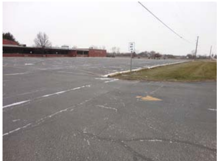
Front Parking Lot
