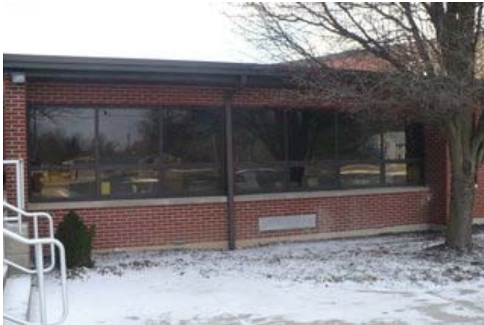
Typical Window of 1959 Addition
