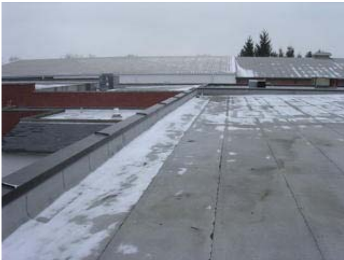
Typical Built Up Roofing
