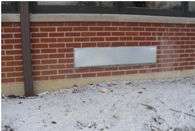
Typical Unit Ventilator Opening in 1959 Addition
