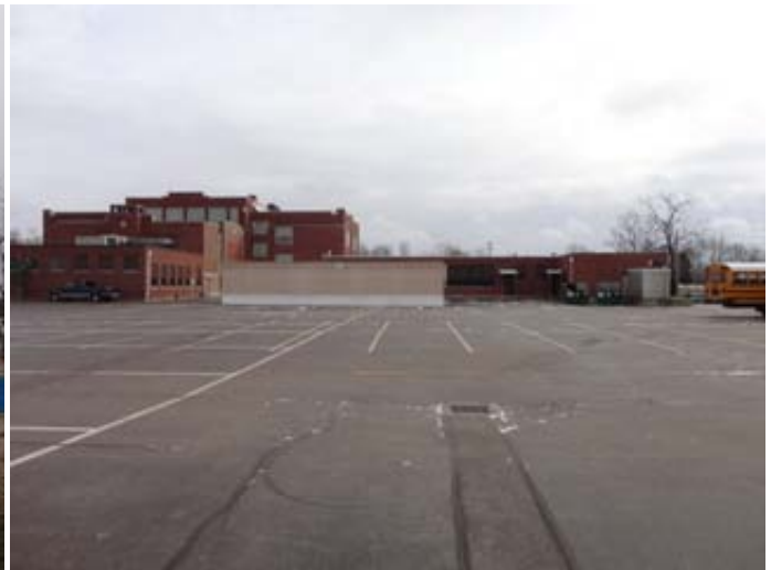
West elevation photo:
