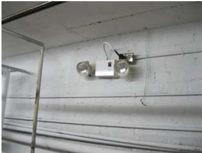
Surface Mount Emergency Egress Light Fixture
