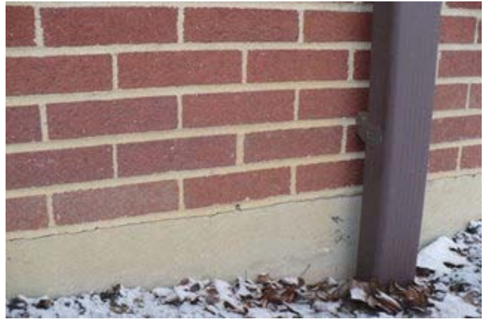
Typical Concrete Base Foundation Wall
