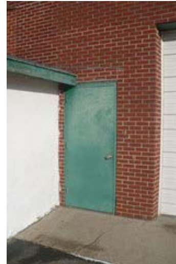
Exterior Door of 1956 Original Construction
