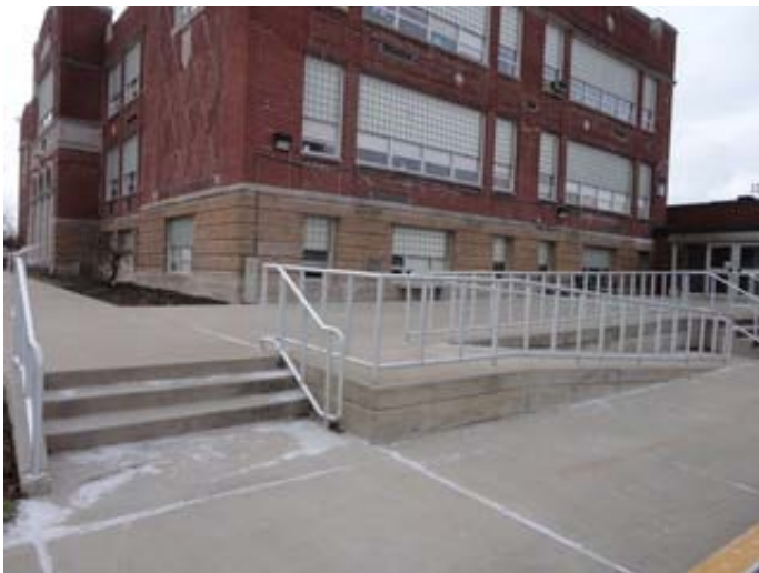
Ramp and Stairs at Entrance
