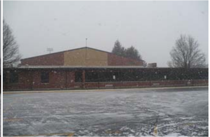
East elevation photo:
