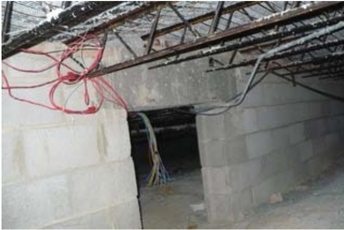
Crawl Space Under the 1959 Addition
