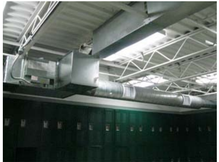
Typical Steel Joist and Tectum Deck Construction in the 1959 Addition
