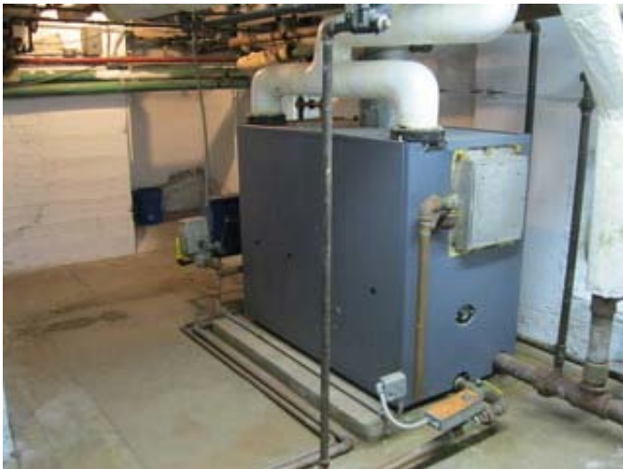
Weil-McLain LP Gas Fired Steam Boiler
