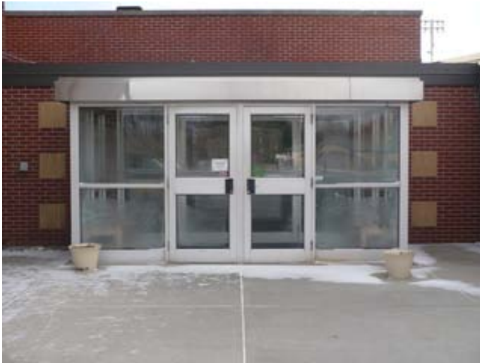
Entrance Vestibule of 1959 Addition
