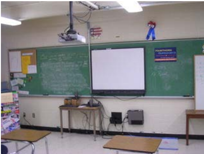
Typical Classroom Smart Board System
